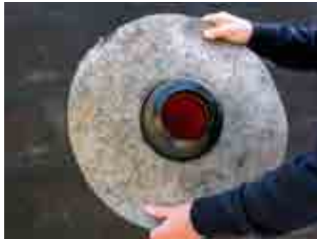
2. Set on bitumen sleeve
