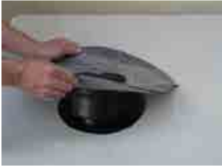
1. Produce tap hole with Ø 255 mm, insert drain HL62H
