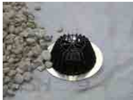
11. Insert leaf catcher, dispense the gravel with minimum grain size 16/32 around the leaf catcher
