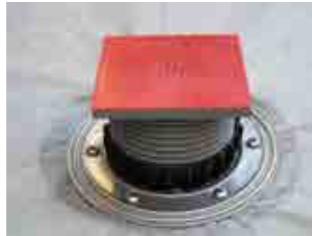
5. Clamp fleece between the stainless steel clamp ring (HL83.0) and the extension (HL85N), set the gravel guard (HL180), adjust the extension to the final slab height
