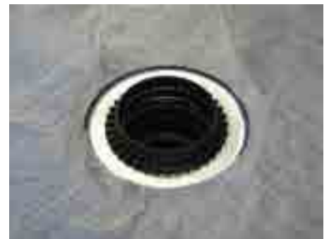
6. Remove lid cover, apply the fleece, insert gravel guard HL160
