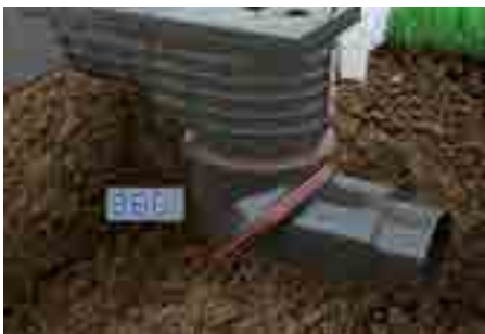
4. Adjust angle to the sewer
